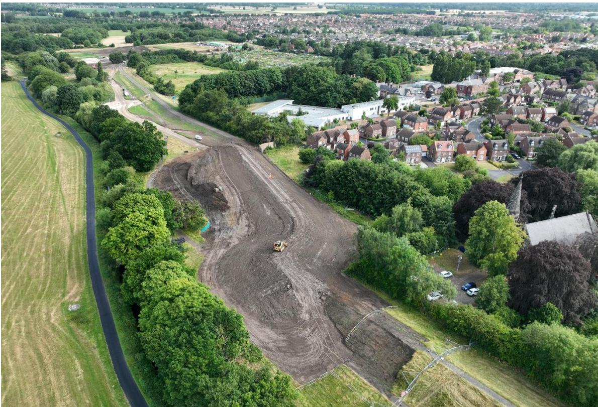
*Photo: Drone footage of the construction of a section of the new embankment, looking northwards towards Rawcliffe Country Park*
